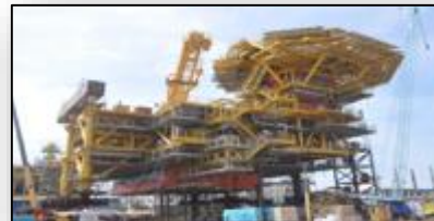
MHSRD III - Topside
