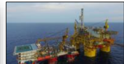
Drilling for Shell Malikai
